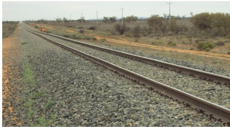
Figure 13: CWR module of 1051.5 km – 1052 km with a steep slope of falling is 1 in 152
